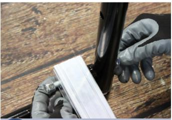
Insert the bolts from the outside of the cart towards the inside. Install a lock nut and tighten down using a socket wrench, but not so tight the handle doesn't rotate.
