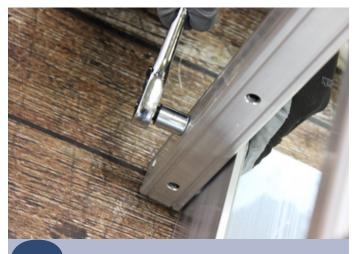
Finish tightening all of the bolts with a 9/16" socket wrench.
